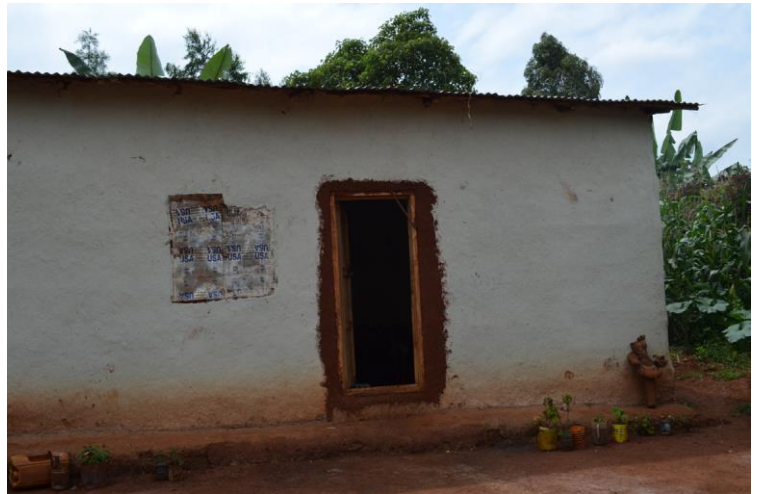
Photo: Workinesh's renovated house
